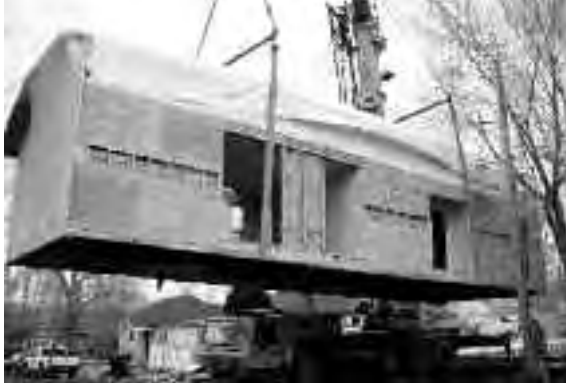
Modular housing being used on infill lots in Magna, UT by Community Development Corporation of Utah.
