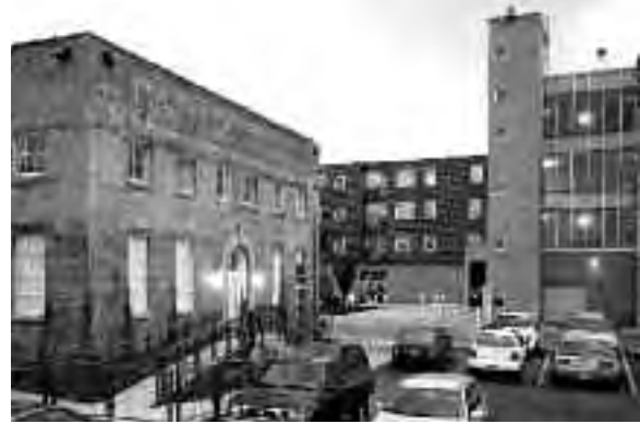
Converted industrial building to live-work space and mixed-use space – Artspace in Salt Lake City
